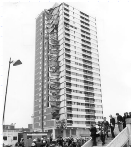
Ronan Point building after May 16, 1968 collapse
