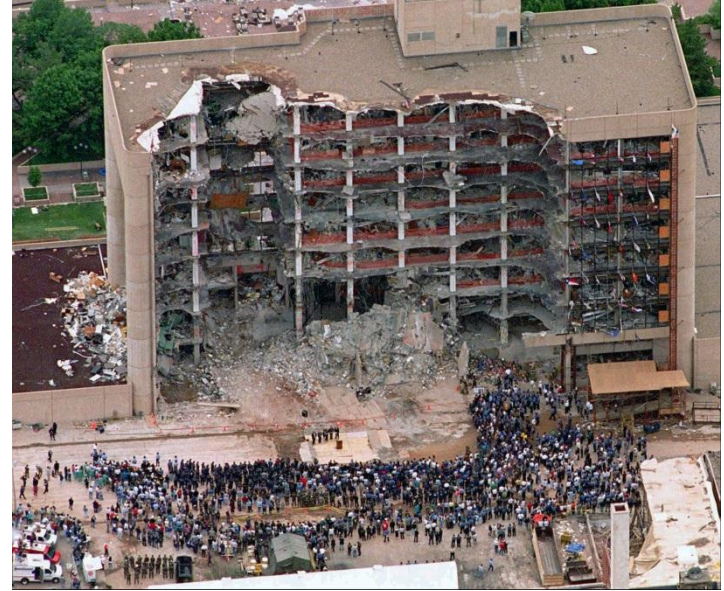
Example of intentional act – Arson, Oklahoma Bomber, USA, Murrah Federal Building before and after. Perpetrator – Mc Veigh. Event leading to progressive collapse. 1995
