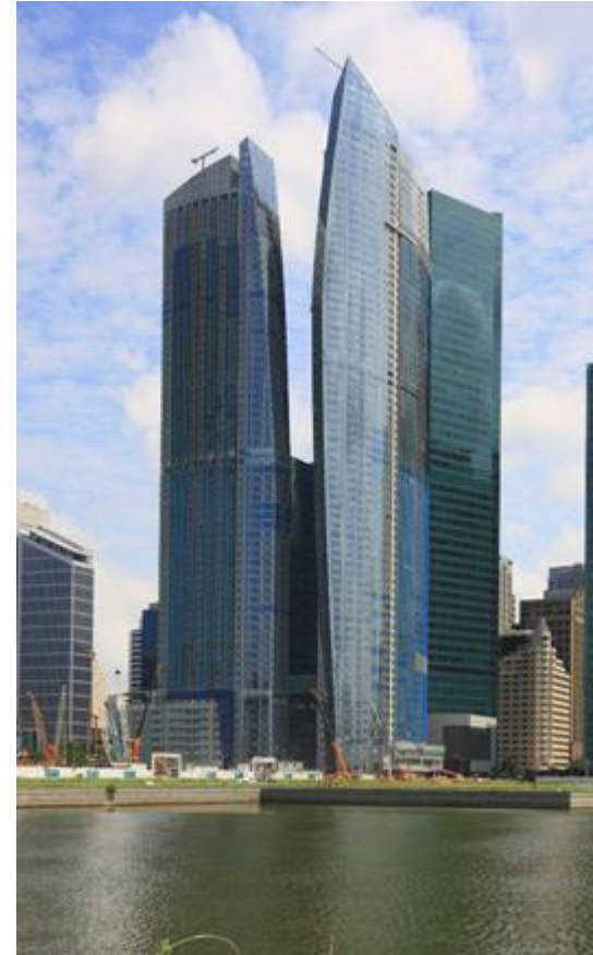
Modern large panel precast concrete structure: The Sail, Singapore
