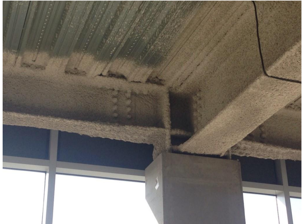
Vermiculite coating to steel structure
