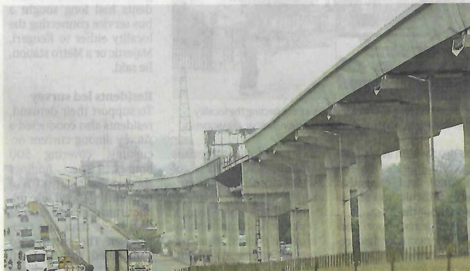
Researchers say the project represents the first corridor-scale techno-economic analysis in India examining direct integration of solar power into a metro rail traction system. FILE PHOTO
